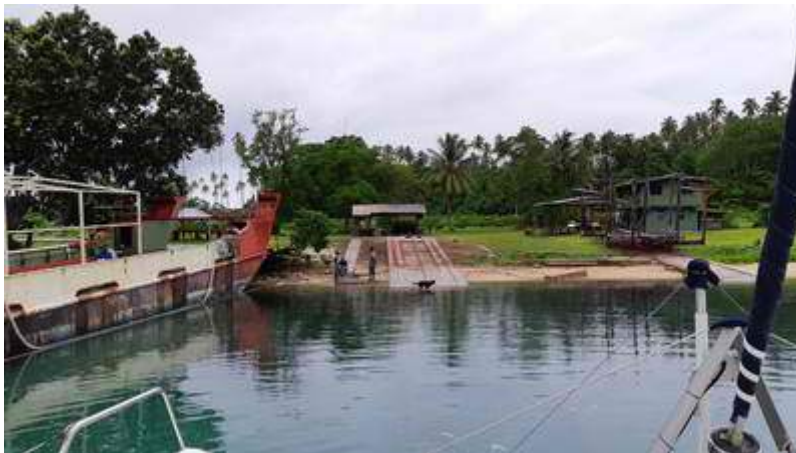
Approaching the ramp with trolley down. The hauling winch house straight ahead
