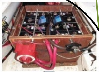
LFP HOUSE BATTERY 540 AHR
